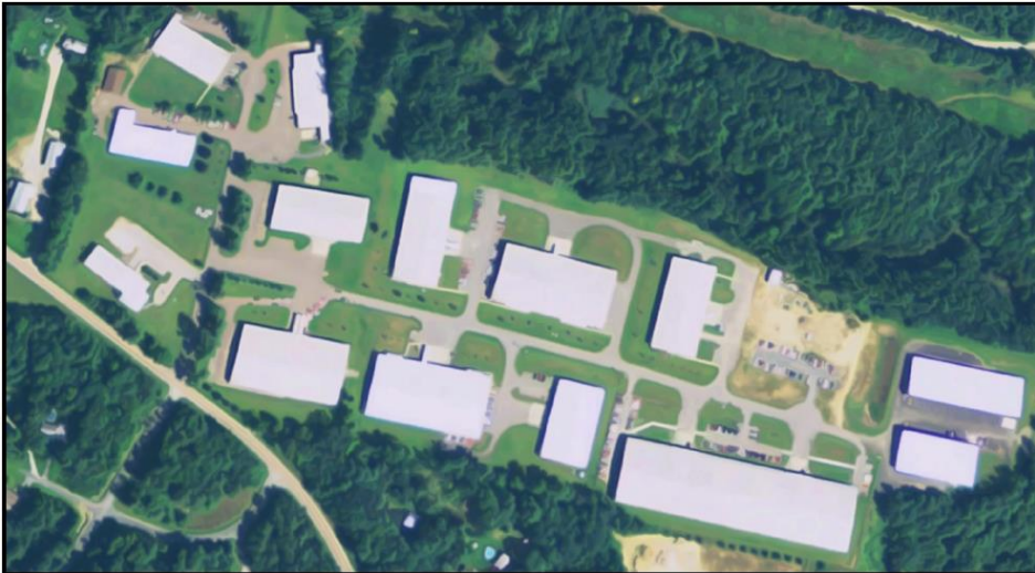
FIGURE 8: Efficient Use – Industrial Example
